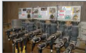
Solid Dielectric Underground Distribution Switchgear
