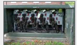
SF6 Underground Distribution Switchgear
